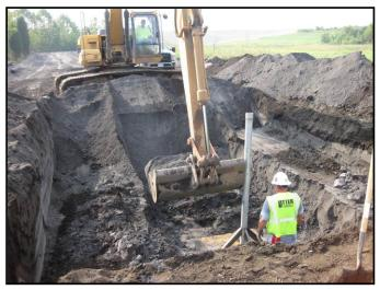
Figure 5A: Settlement Plate Installation
